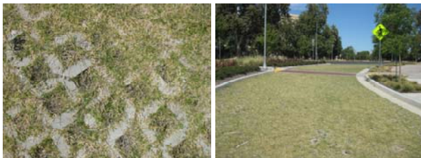
Source: Study OF Chula Vista on Cool Pavement (EPA)
